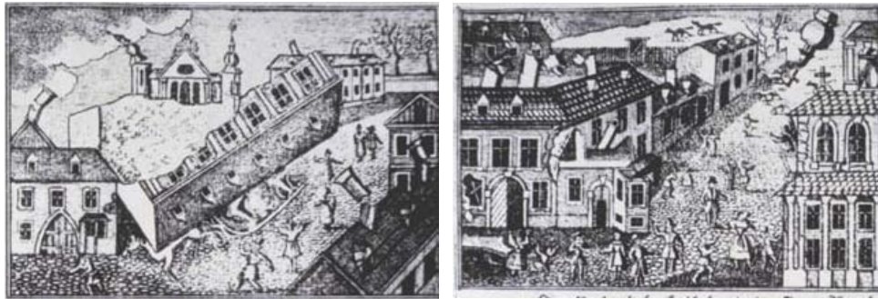
Fig. 3 – Images showing the disaster caused by the January 23, 1838 earthquake (after [16]).
